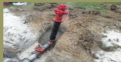
Stand-By Generator at Well #3 and Line Extension with Fire-Hydrant
